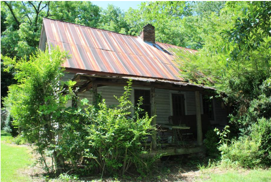
Figure 2 (Former) Johnstone-Hume Slave House
