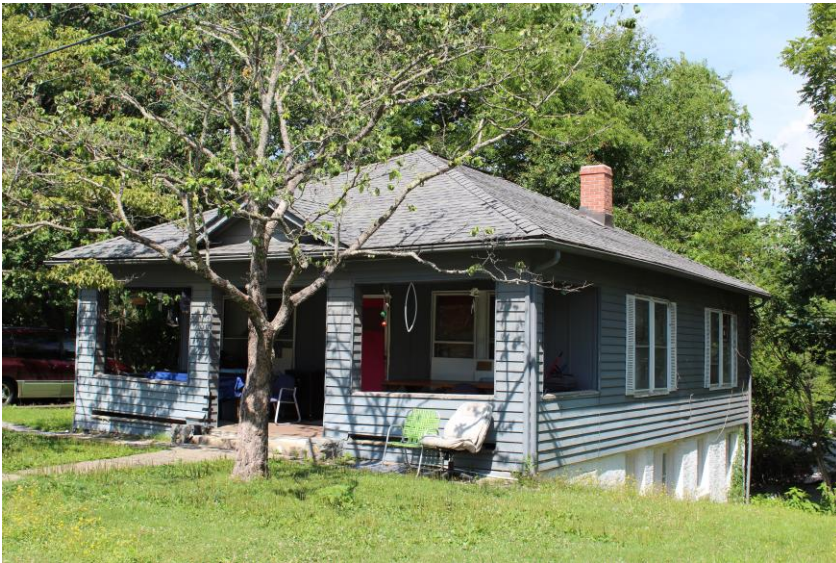
Figure 10. J. F. "Jip" Mills House
