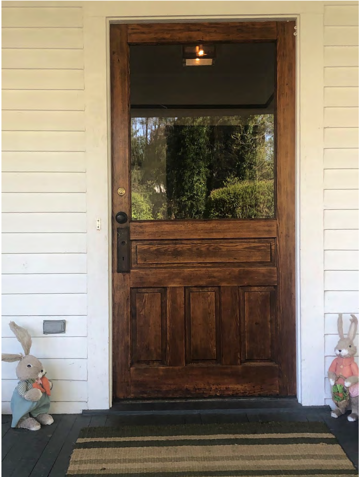
10. Primary Entrance on Front Elevation
